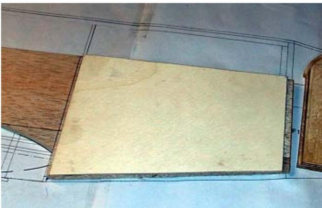
❑ Glue 1/8" front fuse doubler to each side so it will butt against F2 and fit under ledge created by F1A. There should be a 1/4" gap between doubler and front edge of fuse side.
